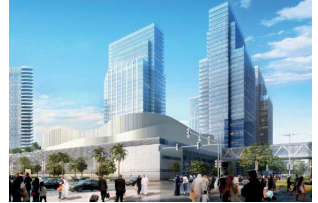
South Overbuild Abu Dhabi
