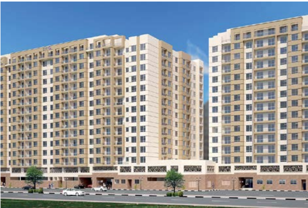
G+P+12 Residential Building Dubai
