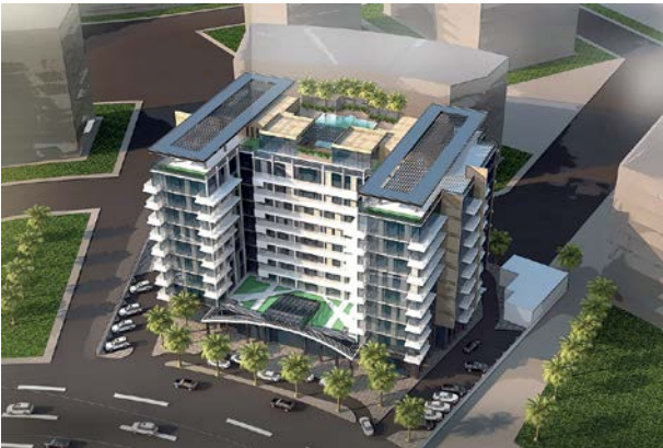
G+8 Residential/Commercial Building Dubai
