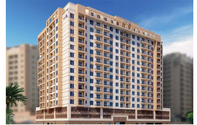
G+2P+12 Residential Building Dubai
