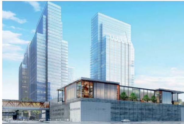
North Overbuild Abu Dhabi
