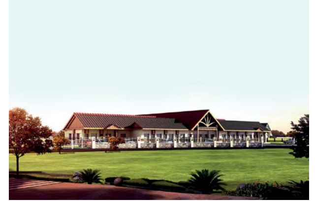
Khalifa Bin Zayed Al Nahyan Hospital Perseverance Island, Seychelles
