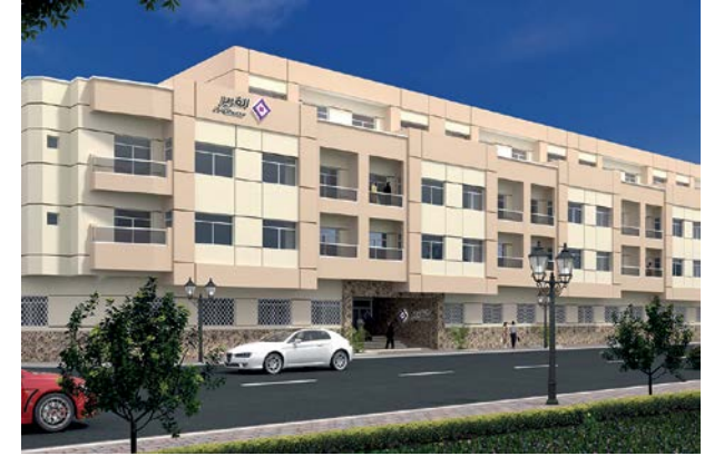
2B+G+2 Residential Building Dubai
