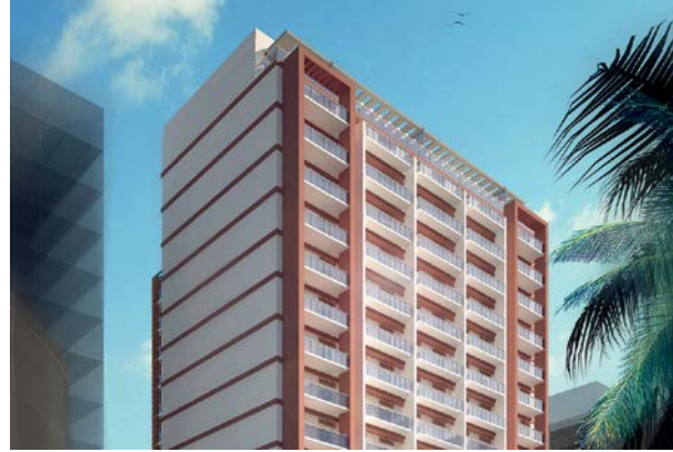
G+16 Mixed Use Building Dubai
