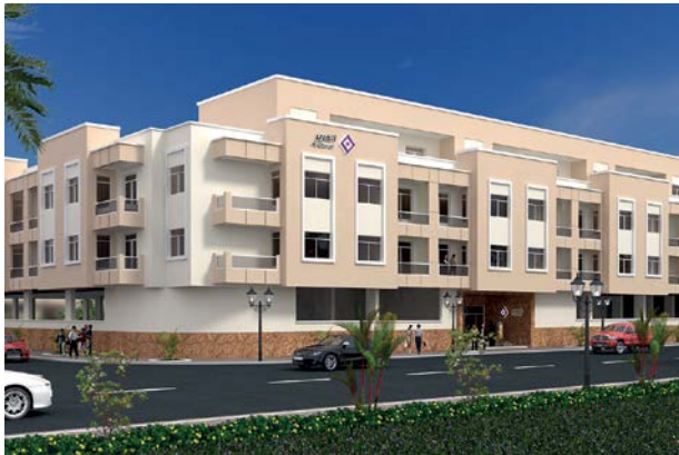
G+2 Residential Building Dubai
